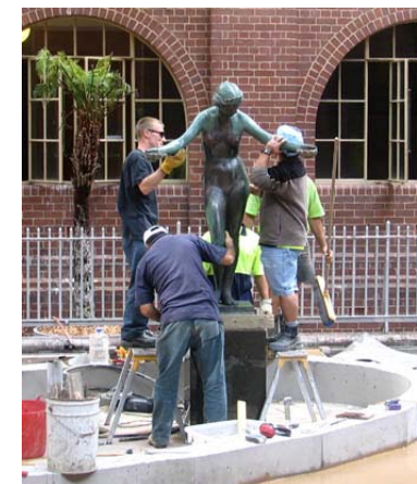
Re-installing the Naked Lady
